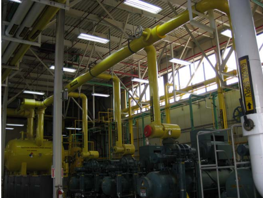
Photo of Building 62 after the Lighting Retrofit.
